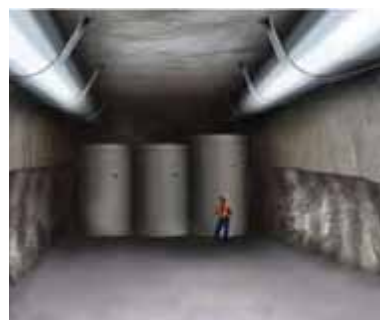
3: Resin Liner Shields within ILW emplacement room
