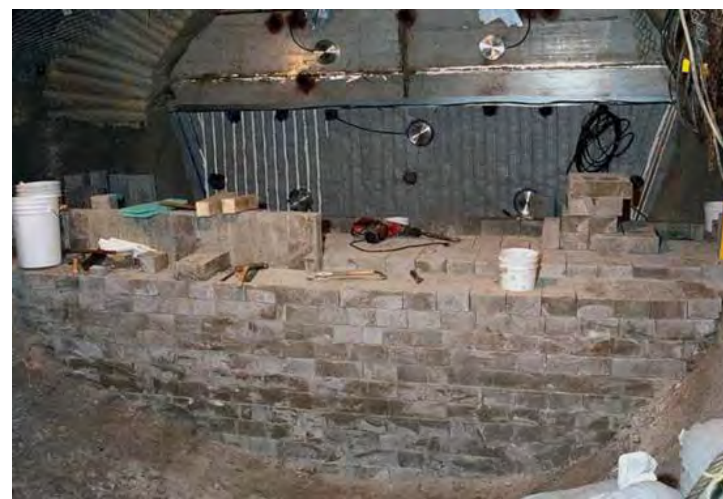
Precompact Bentonite Blocks
