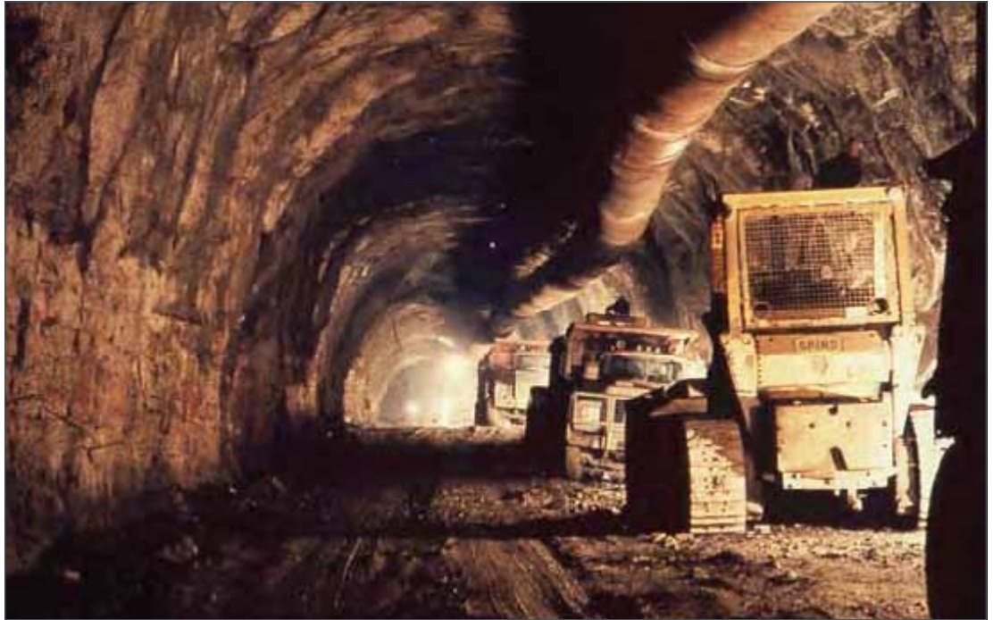
Darlington cooling water intake tunnel
