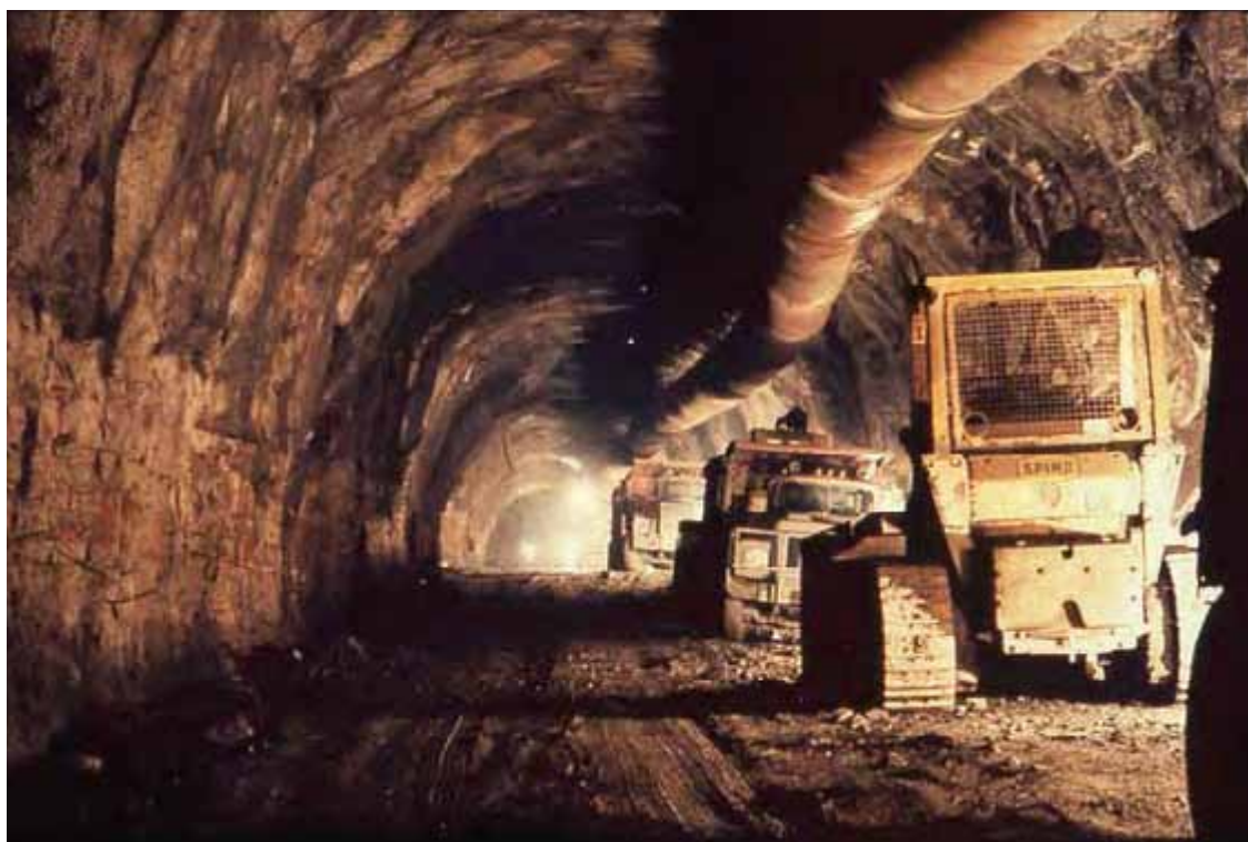
Construction during Darlington cooling water intake tunnel
